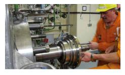
In a German power station, the shafts of the main feed pumps are sealed with EagleBurgmann type **DF-SAF1/165** mechanical seals with DiamondFace coating.
