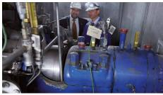
The EagleBurgmann **DF-SAFI4/188** diamond-coated mechanical seal runs in the boiler feed pump of the black coal power station in Voerde, Germany, to the complete satisfaction of the operator. Operating conditions: p = 21 bar (305 PSI); t = 158 °C (316 °F); n = 5.100 min<sup>-1</sup>.
